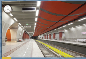
Work completed at the Athens Underground
